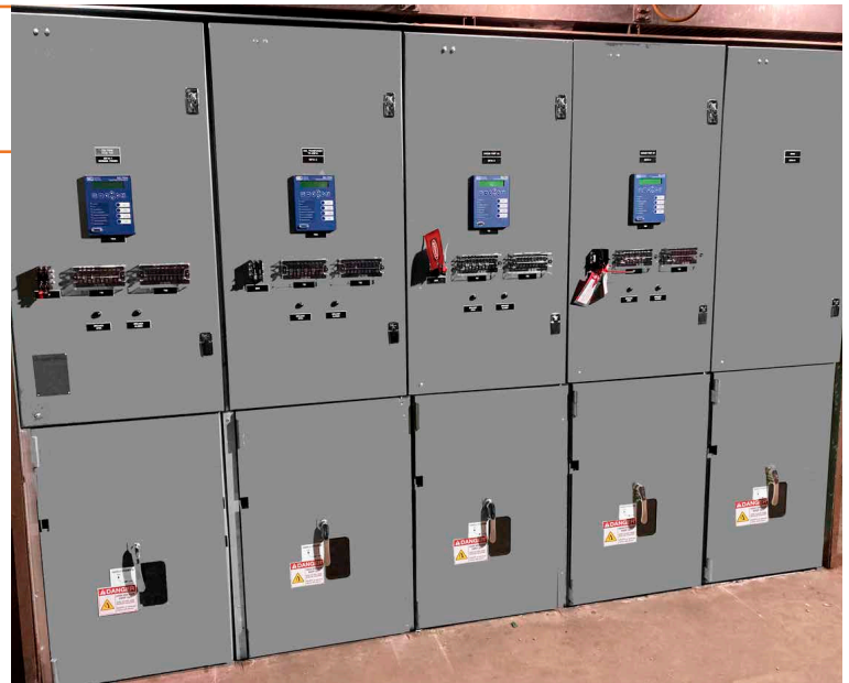
Pictured here is the team's design and installation of a 5KV line-up of older vertical lift GE-AM breaker retrofits with horizontal roll in PowlVac circuit breakers.
