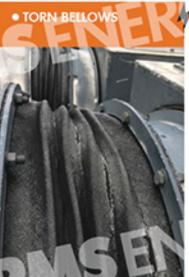
Torn and improperly installed rubber bellows allow moisture and contaminants to enter the bus system, causing damage and risking major repairs.
