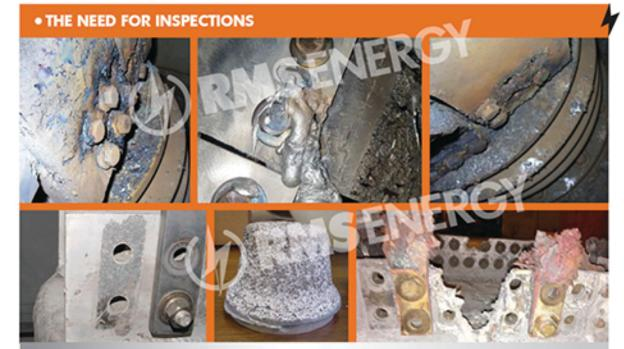
Often, plant maintenance programs make an incorrect assumption that IPBD systems are self-maintained with little human intervention needed. However, IPBD systems should be treated with utmost importance, being inspected, cleaned, monitored, and maintained on a regular basis for optimal performance.
