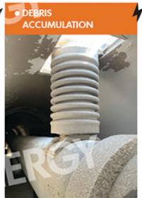
Dust and other forms of intrusive debris can become conductive and will act as a sponge when exposed to moisture, degrading insulation integrity and leading to damage.
