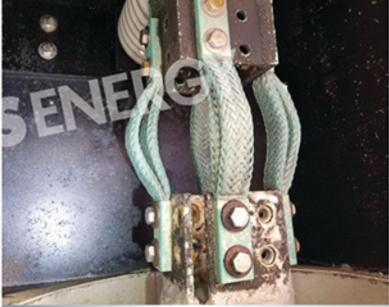
Moisture accumulation in cracks or fissures can result in phase-to-ground faults.
