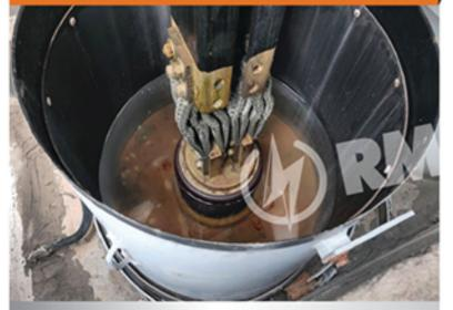
Moisture is by far the most common cause of bus system failures. Corrosion and damage to heaters and other components can lead to major repair and costly downtime.
